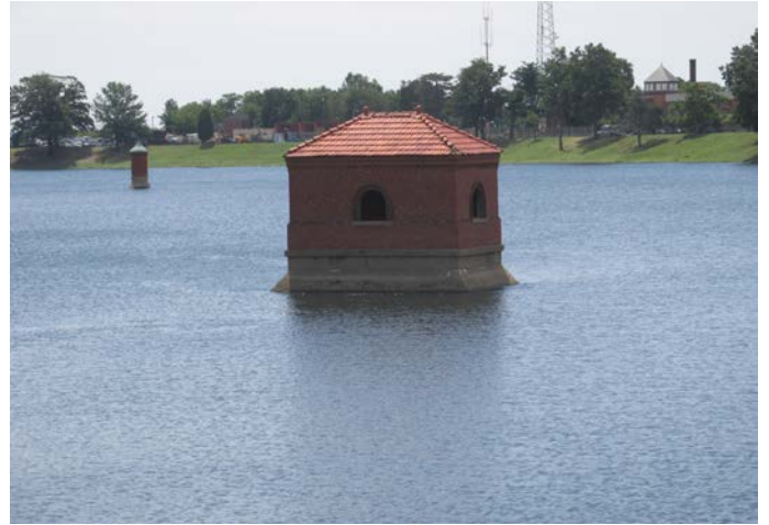
Circulating Conduit Building in the McMillan Reservoir
