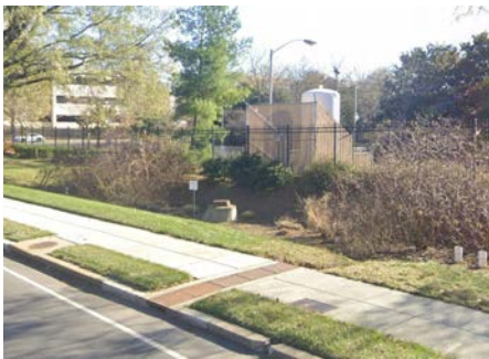
Bio-retention on Irving Street
