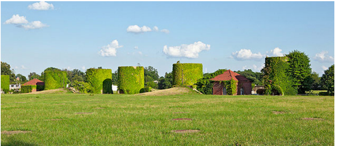
The McMillan Sand Filtration System
