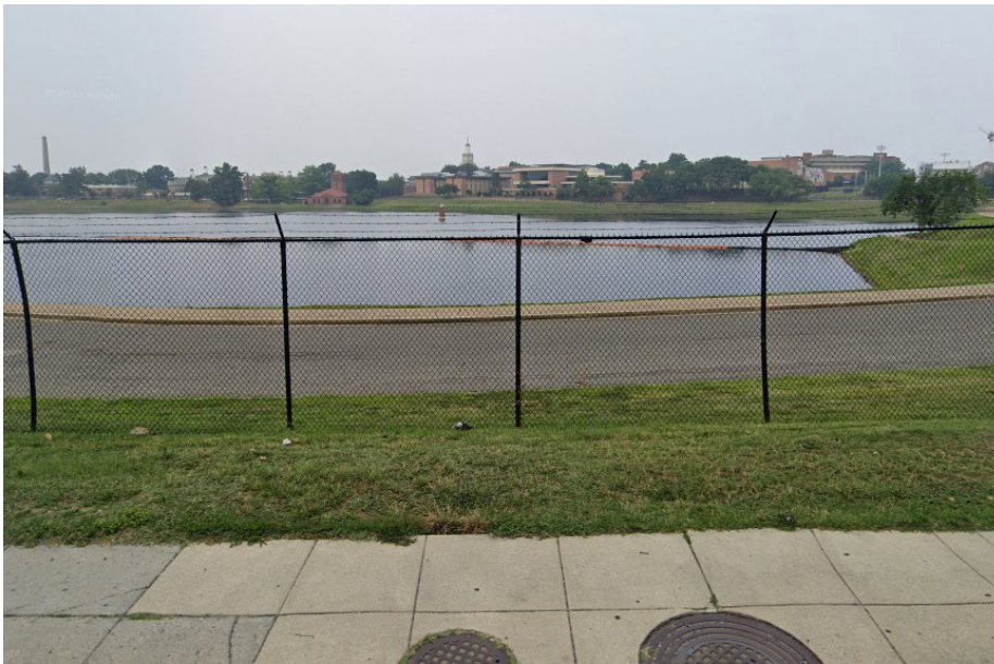
McMillan Reservoir Fencing
